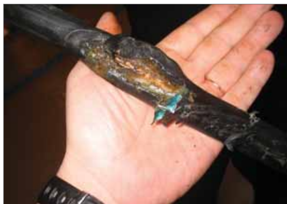
Figure 7.2: Cable damaged by fishing gear. A grapnel intended to retrieve fish traps from 1,800 m depth damaged the insulation and fibres on this cable. Source: Tyco Telecommunications (US) Inc.
