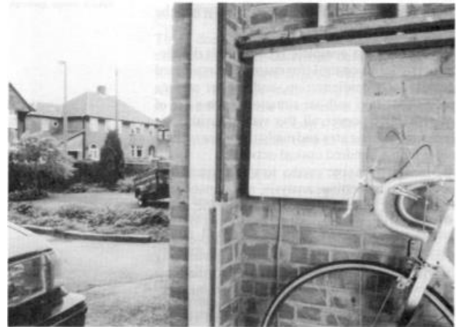
Figure 8—TPON network termination
