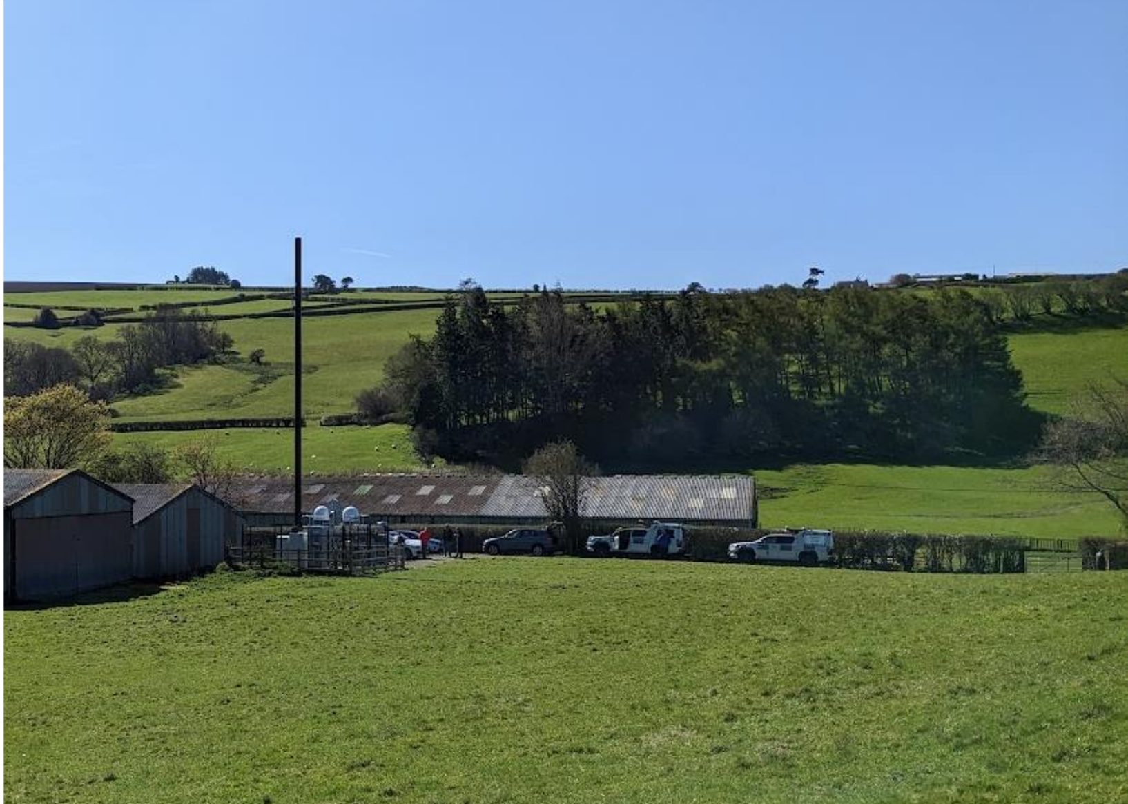
Extremely rural connectivity - GEO satellite backhaul
